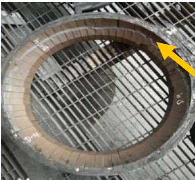
Erosion due to Coal Roping
